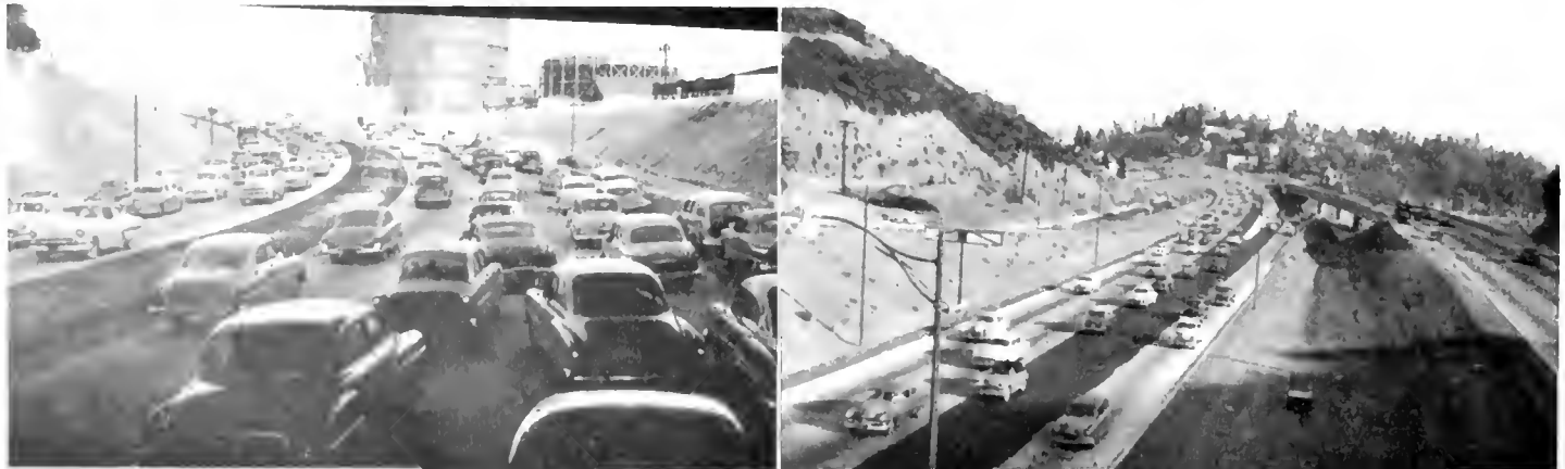
LEFT Looking easterly along completed Santa Ana Freeway from under Alameda Street Bridge, showing late afternoon peak traffic. RIGHT View looking south-easterly along completed Hollywood Freeway showing late afternoon peak traffic at junction with inlet ramp for outbound Highland Ave. traffic. In background is fine residential area known as "Whitley Heights" and off the photograph to the right is the Hollywood Bowl.
